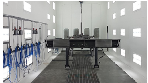
Concrete Pit Installation
