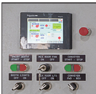
Optional UL/CSA listed control panel with or without VFD
